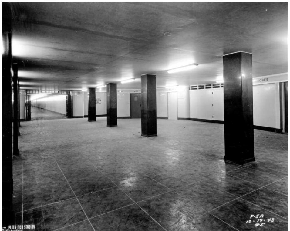
quarter of an inch thick. The terra cotta was delivered in pieces 11-inches by 22-inches and laid in a manner similar to that described for structural glass.
